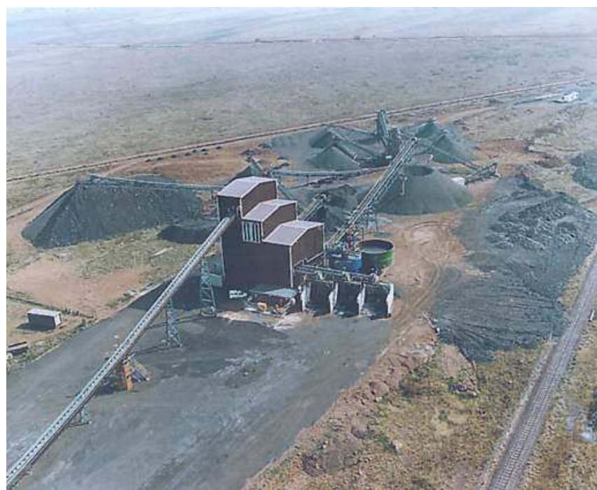
Figure 5 : 1,5 million tpa Metal From Slag Recovery Plant
